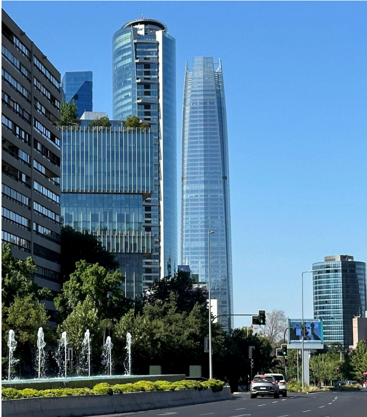
Figure 2 - 62-story skyscraper Gran Torre Costanera in Santiago, Chile
