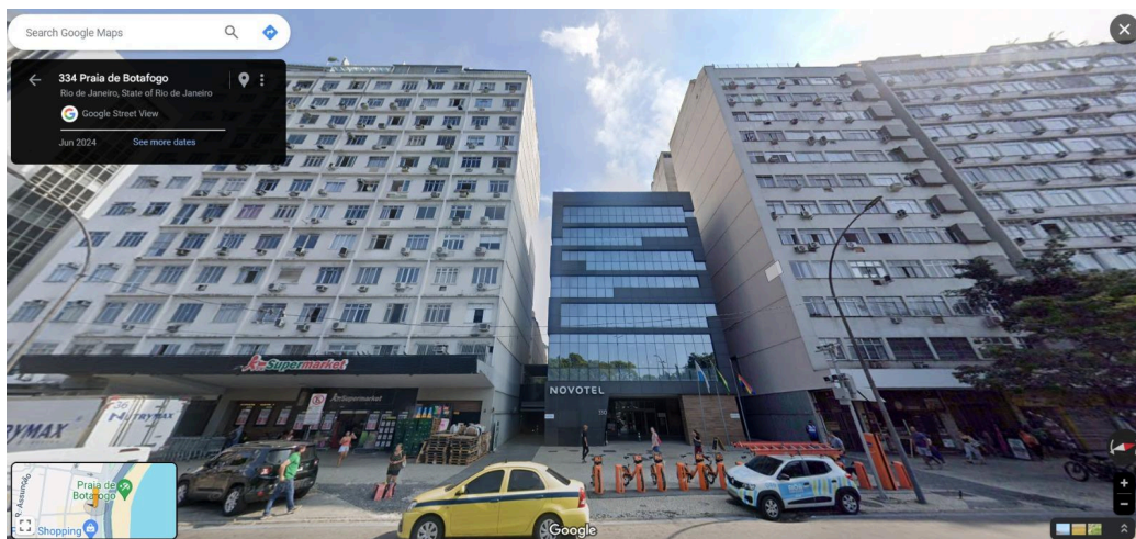
Figure 14 - Novotel Botafogo on building restrictions
