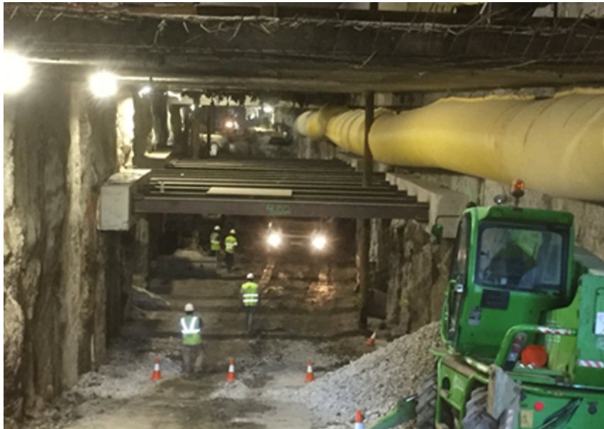
Figure 3- Subway works (@Martim Smolka)
