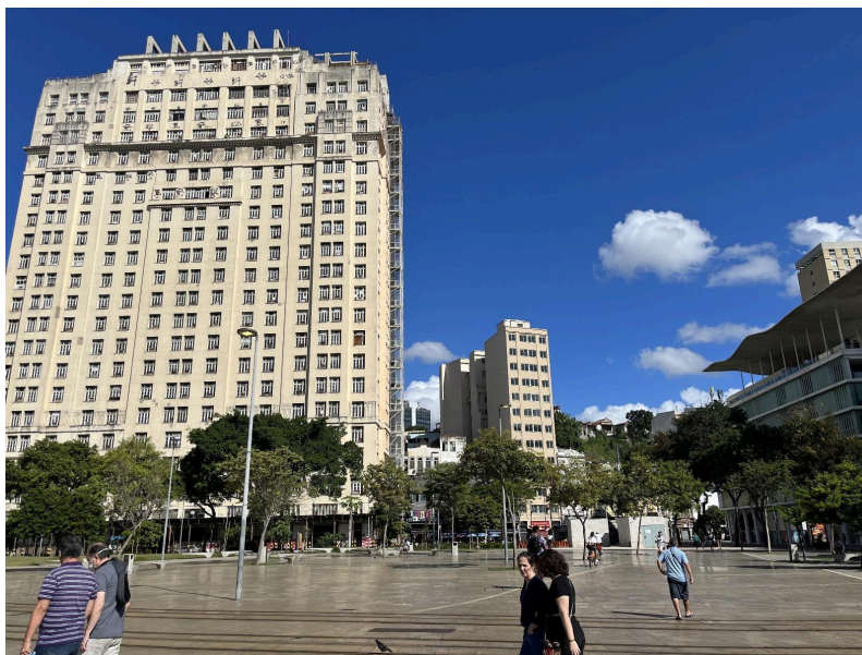
Figure 16 - 'A Noite' building refurbished under Reviver Centro
