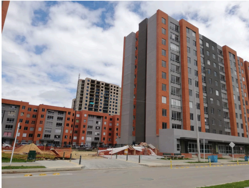
Figure 20 - Partial Plan Lagos de Torca - Overview of the project (@Maria Cristina Rojas)
