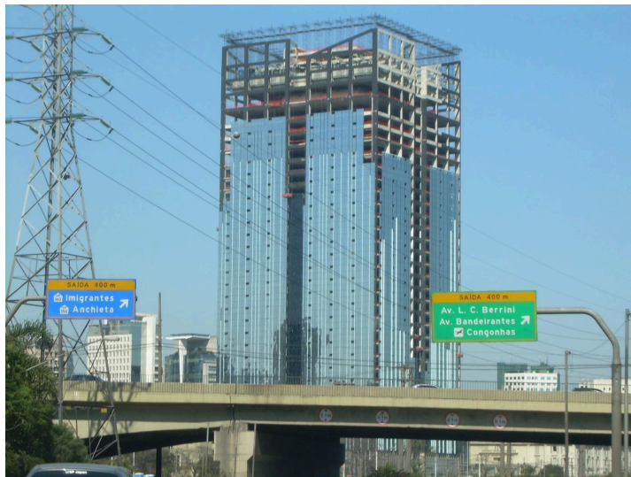
Figure 11 - OODC charged in building in São Paulo
