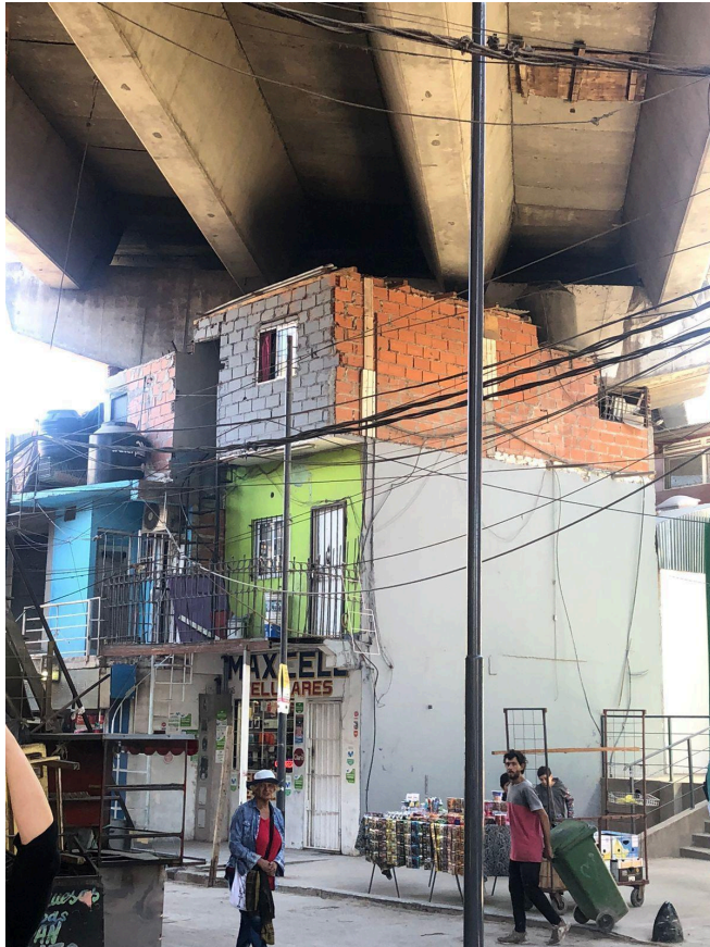
Figure 55 - Limits to additional building area limits may be physical... Buenos Aires Vila 31
