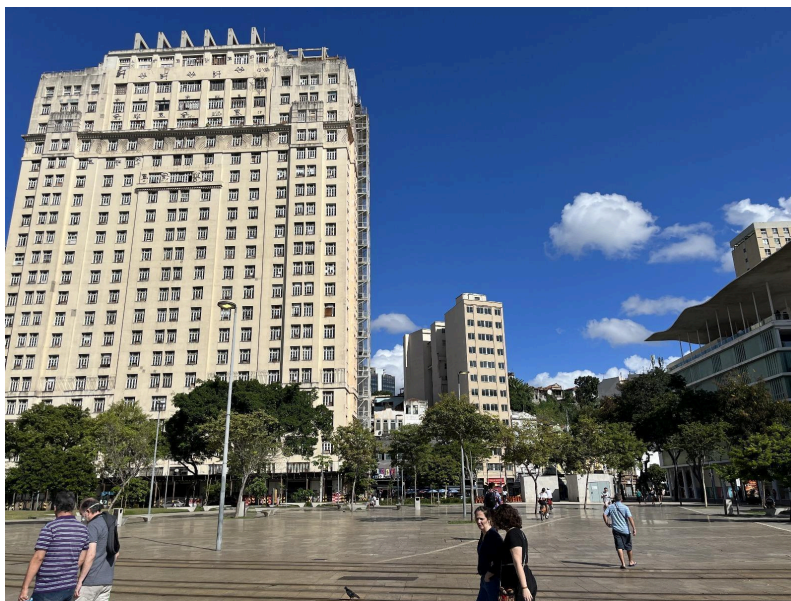
Figure 16 - 'A Noite' building refurbished under Reviver Centro
