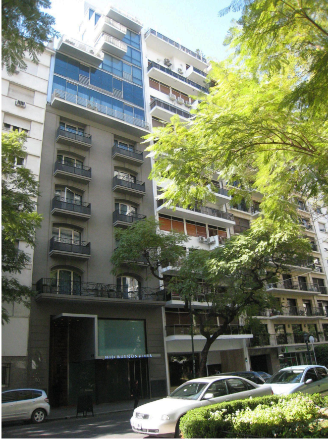
Figure 30 - Added new area in an existing building in high end Ricoleta neighborhood. (@Martim Smolka)
