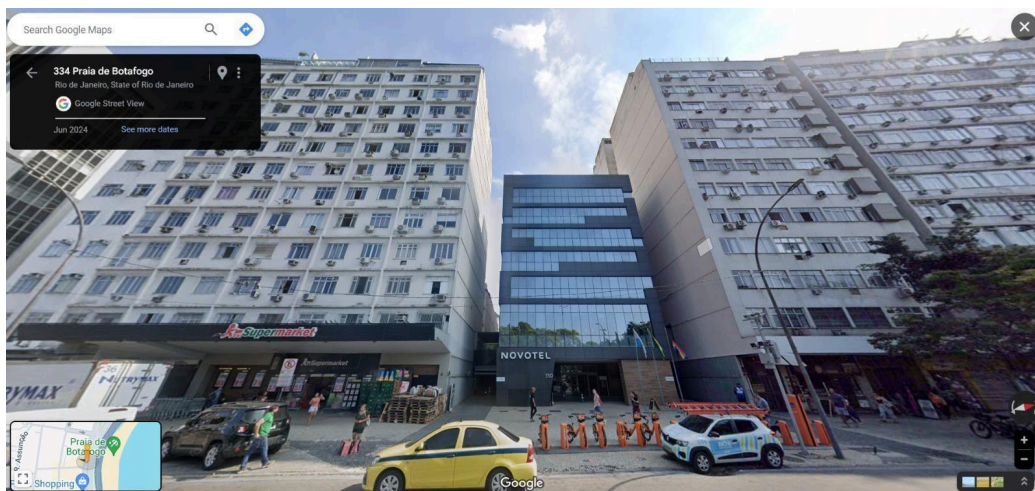
Figure 14 - Novotel Botafogo on building restrictions
