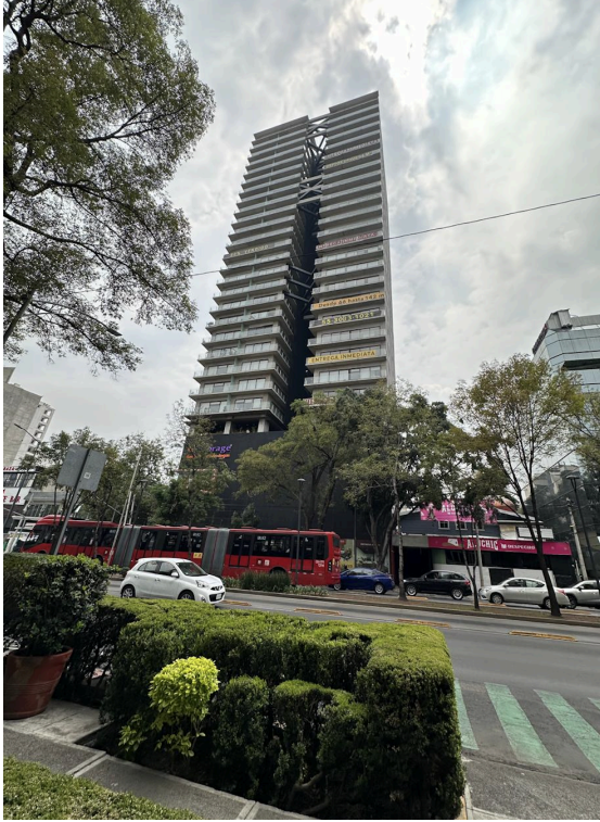
Figure 34 - Building benefitted by transfer of building rights in Ave. Insurgentes Sur 1831 and 1857 (@Salvador Gómez Rocha)
